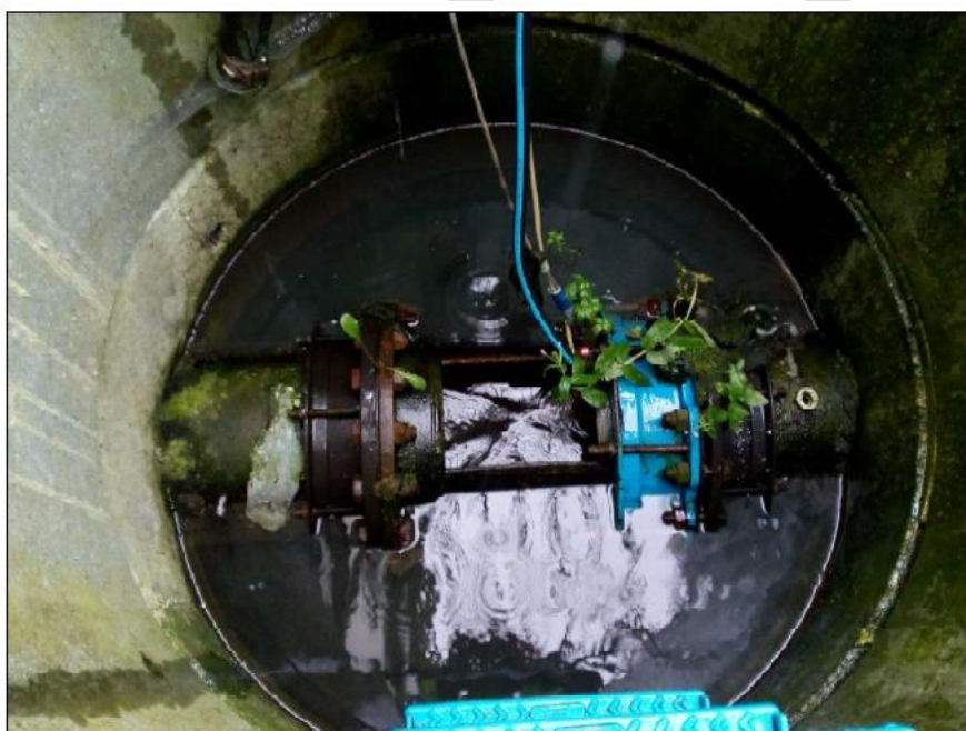
Figure 3-37: Moycullen final effluent area velocity meter
